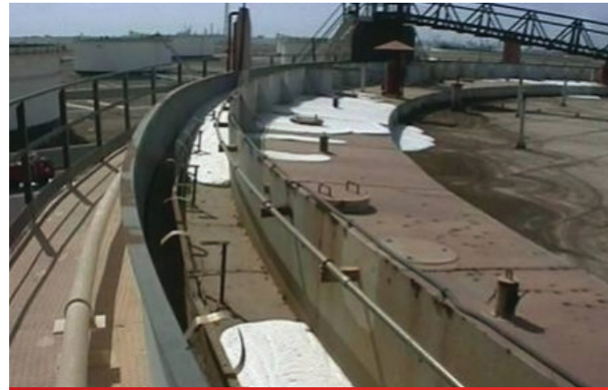
Too rich proportioning, meaning the foam solution cannot flow effectively to seal on a tank rim seal test (image courtesy of LaStFire)
