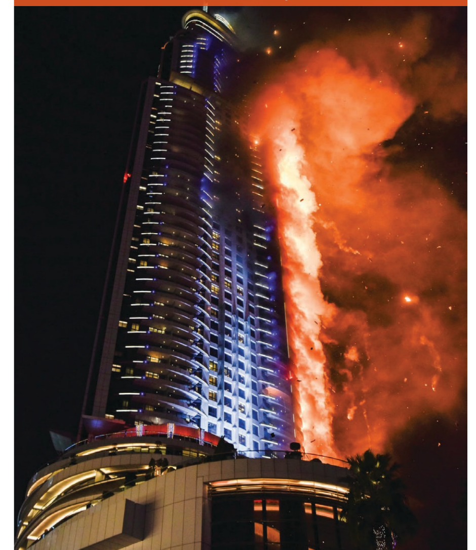
High-rise fires present unique challenges due to the height of the building, the potential for rapid fire spread and the need for effective evacuation and rescue operations
